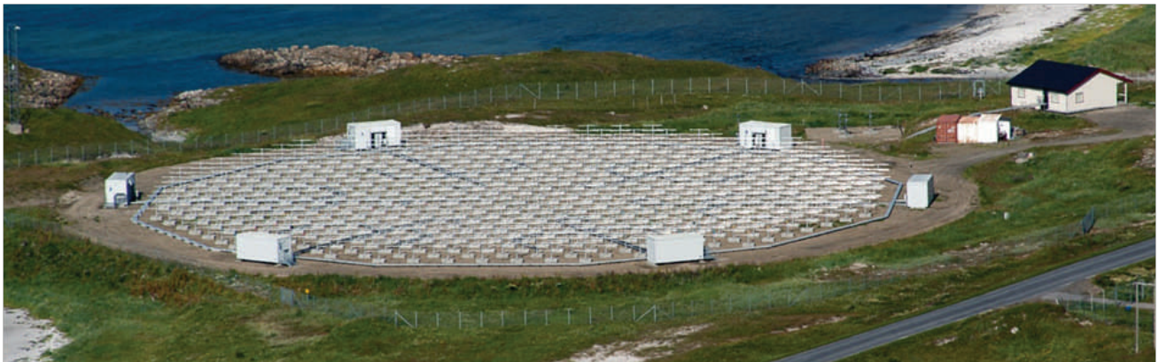
Figure 1. View of the MAARSY site in July 2011 showing the main antenna array, the six equipment buildings at the perimeter of the array and the main building housing control and data acquisition hardware.
